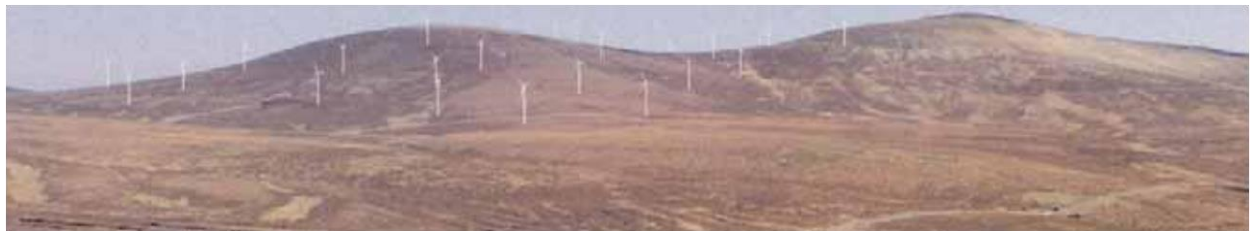
1(b) Wind energy development with many turbines of medium height – this can be inappropriate. The spatial extent of a wind energy development can be reduced by using taller turbines. This may be a preferable solution in some situations.
